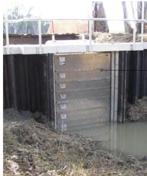
An aluminium and stainless steel, customised regulator was manufactured for easy wetting and drying of the lagoon.
