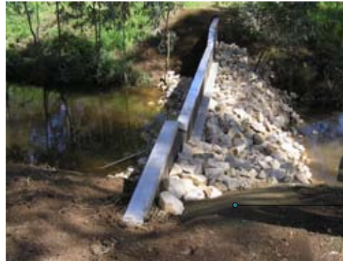
Geofabric to protect against soil erosion.
